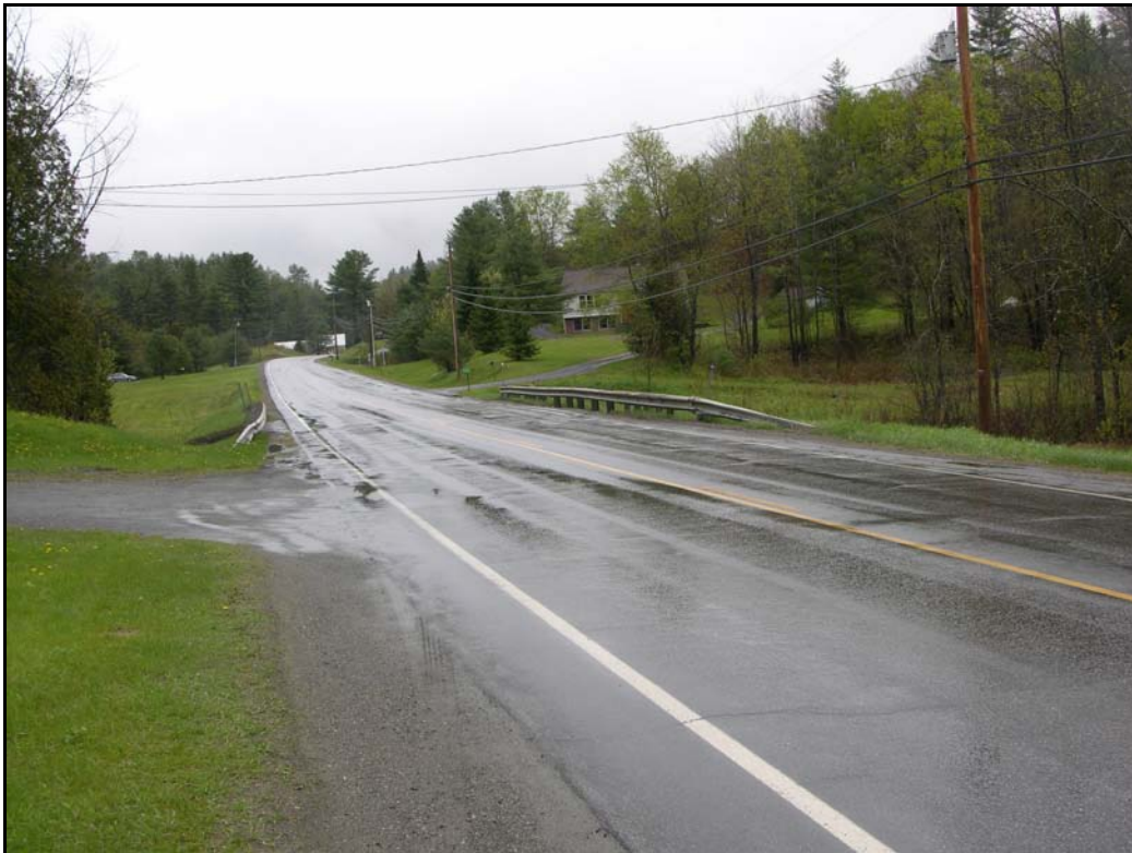
Figure 1: VT 14, Bridge 82 over Kingsbury Branch River
