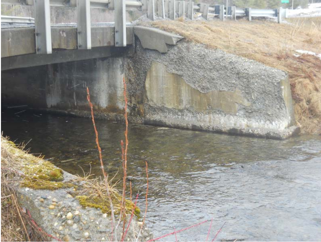
Spalling on a wing wall.
