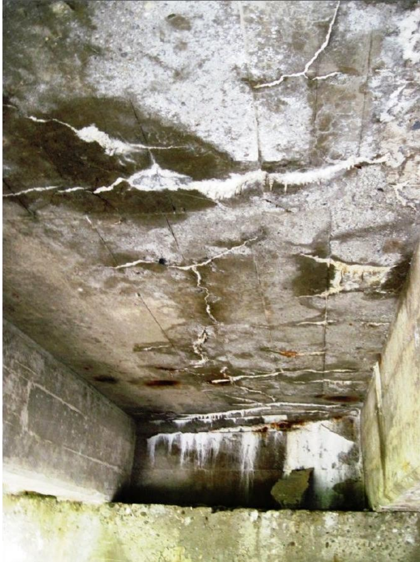
Cracking in the underside of the deck.
