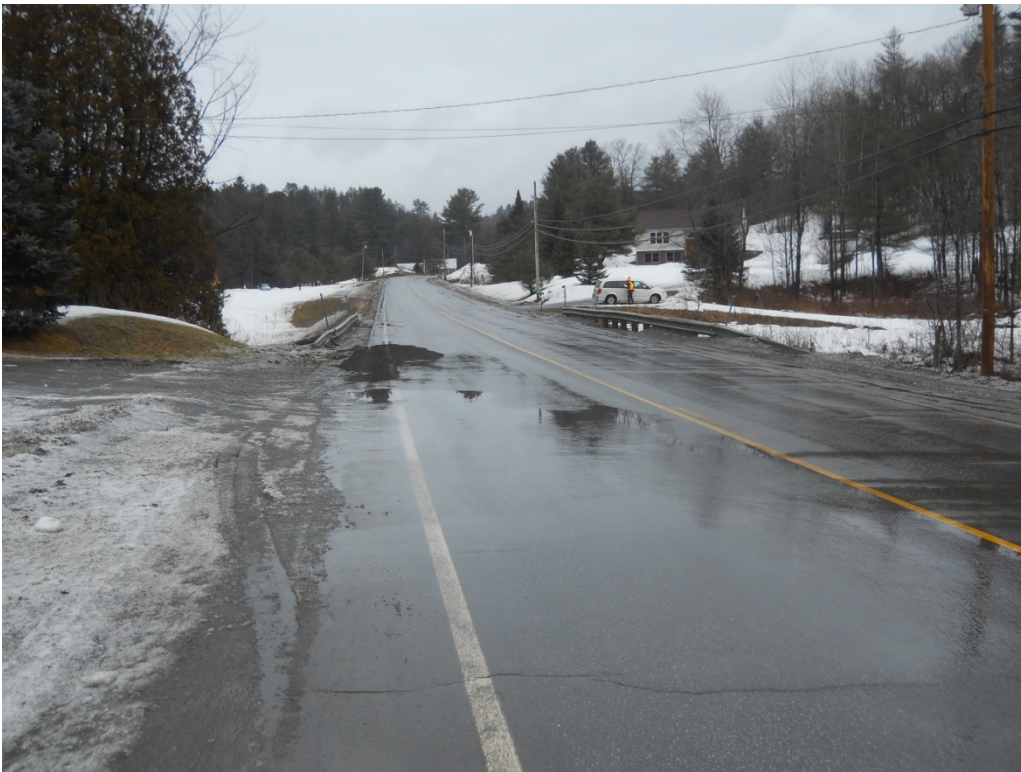
Looking to the north.
