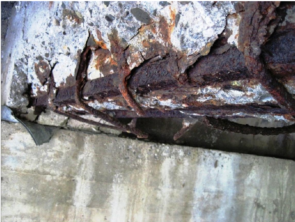
Exposed reinforcement on the T-beam superstructure.
